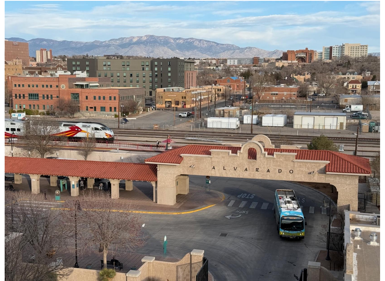
Alvarado Transportation Center
